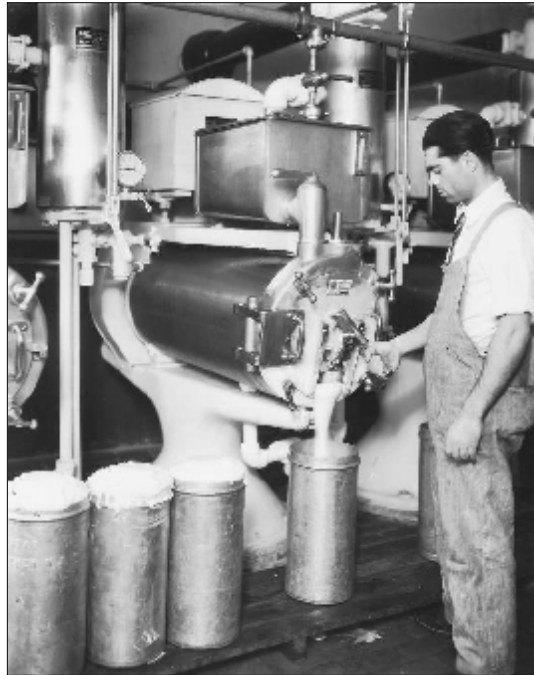
A Costa's employee using the Direct Expansion Freezing Machine, ca. 1928. This is one of the many photographs donated to the Society by Gregory Costa.
